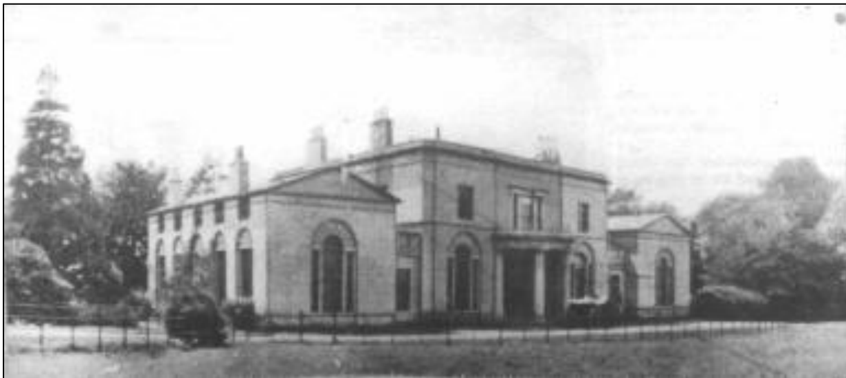
Figure 4. Chessel House. Photograph c.1915
