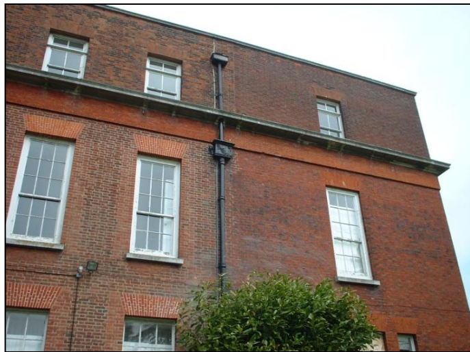
Figure 3. South Stoneham House, drainpipe on south front
