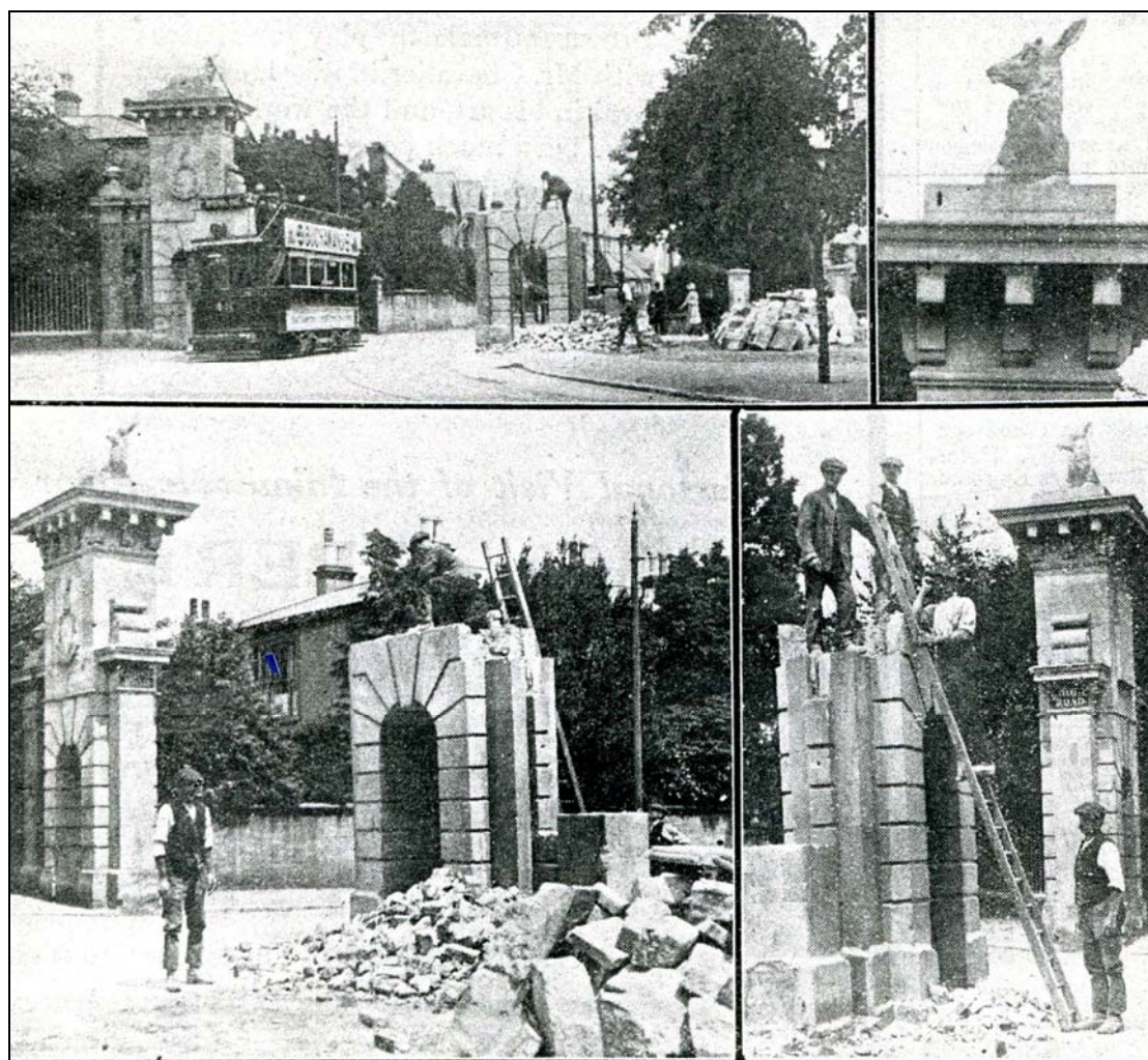
Figure 3. Photographs of the demolition of the Stag Gates from the Southampton Pictorial , 17 June 1919. (courtesy of Brian Ticehurst)
