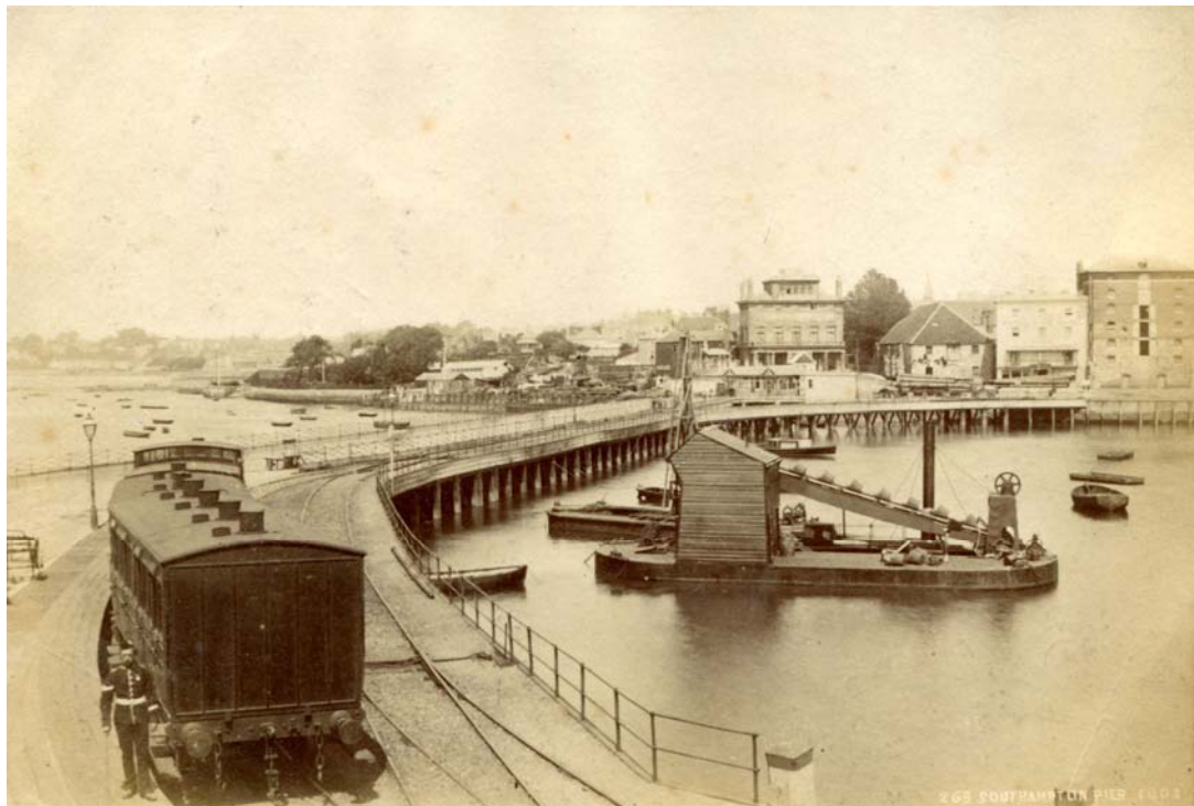
Figure 5. From the 1880s, note the alterations for steam hauled trains; additional track to allow a runround facility, the extra pier structure to provide direct access, and the single storey entrance building.
