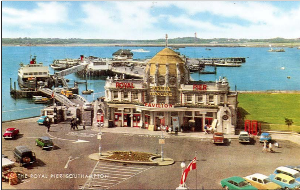
Figure 19. The pier is by-passed by cars though passengers still board via the pier circa 1965. It will not be long before new facilities remove all trade from the pier.
