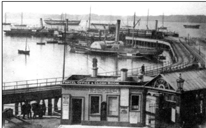
Figure 6. An 1880s view clearly showing the separate structure for the railway line and some of the entrance building.
