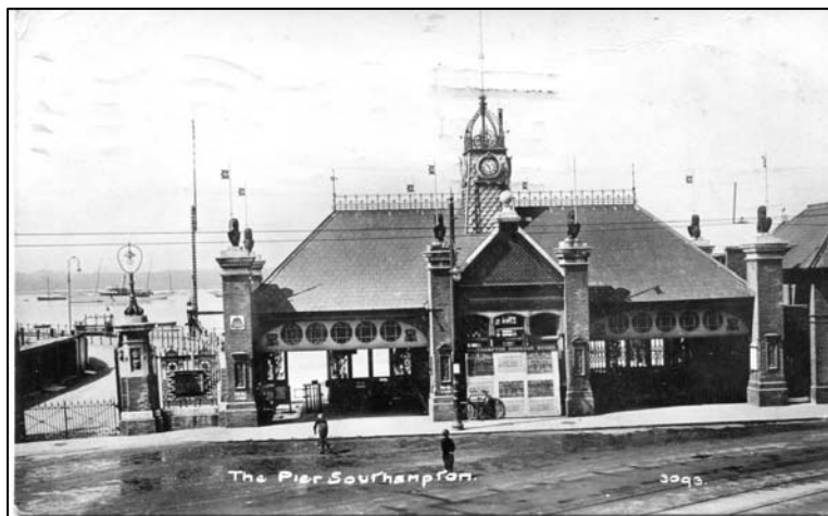
Figure 11. Townside of the 1892 entrance. A post 1911 view as the tram tracks have arrived
