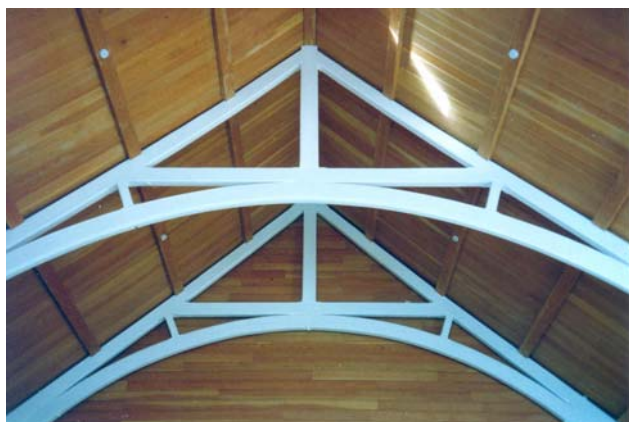
The glued laminated timber arches in the schoolroom designed by J.G. Poole in 1860, now the Marriage Room of Southampton Register Office (photograph courtesy of Dr L.G. Booth and Diana Heywood).
